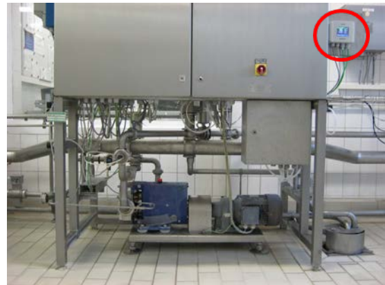
Picture 2: Example of yeast dosing. Whereas the two TurbiGuard sensors here cannot be seen, the control unit SICON M is encircled.
