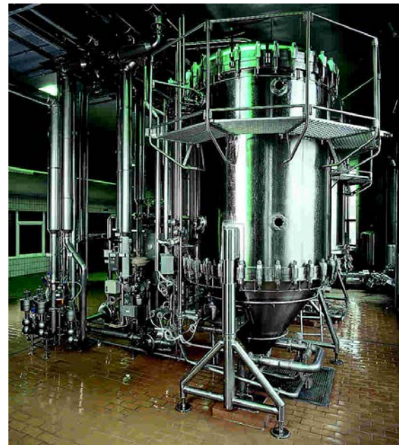
Picture 2: Typical Kieselguhr filtration plant
